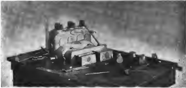
Aluminum Cylinder Pattern and Tools Used In Making.
